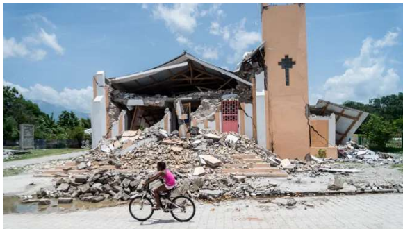
Damage to a church in Haiti
