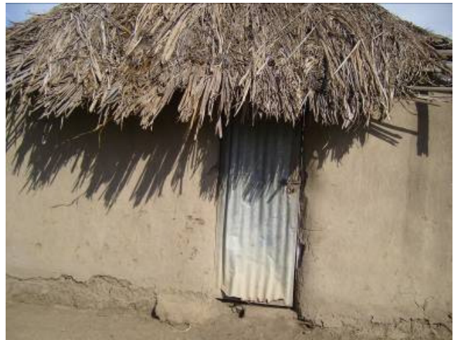
A typical house in Kadibo Division – Kisumu
